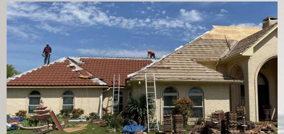
Roser Terracotta Cleo Barrel tile, installed direct to deck, replaces concrete tile installed on spaced sheathing...
