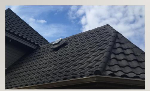
Roser Charcoal Cleo Barrel tile replacing hail damaged synthetic slate look ...
