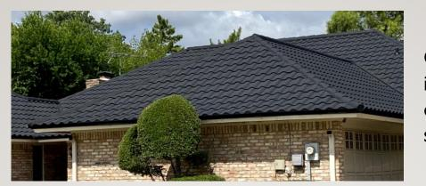
Cleo Charcoal Tile installed over Hail damaged composition
