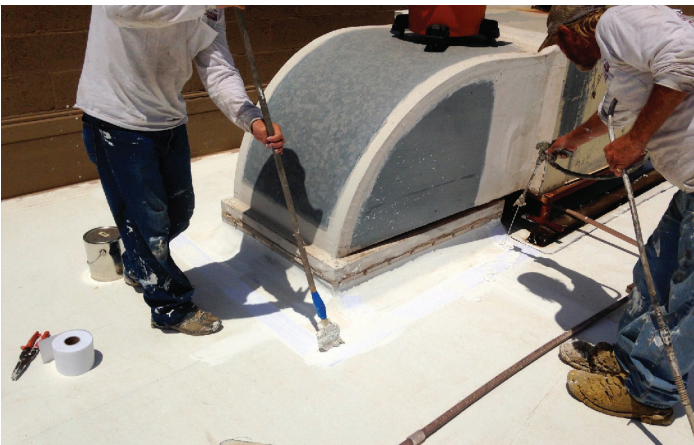
Karna-Flex WB applied to TPO with spray equipment
